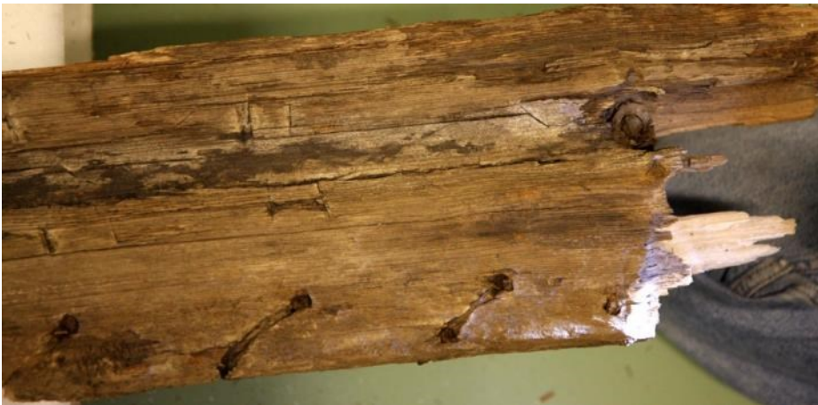
Planks. Detail with sewn planks.
