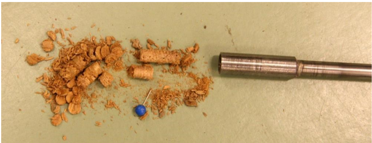
Not all the cores came out in one piece. This is an example where the interior of the item is completely degraded.
