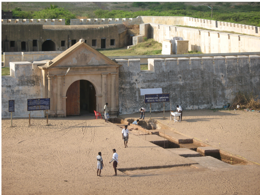
Fig. 2. The excavation revealed important traces of the original drawbridge over the former moat around Fort Dansborg as well as several daily life objects such as clay pipes, Chinese porcelain, European wine bottles and Indian clay pots, and the items found testify to the profound material cultural exchange locally and internationally. Photo: Nils Engberg, 2007. (National Museum of Denmark).
