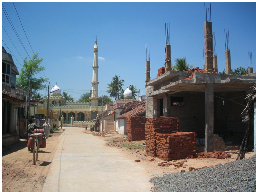
Fig. 25. Construction of a new house in Mosque Street. The Muslim community in Tranquebar has a longstanding tradition of male work migration to Arabic countries and Southeast Asia, and building a new house with the earnings made from the work signals the financial success of the owner. Text and photo: Helle Jørgensen, 2008. (National Museum of Denmark).
