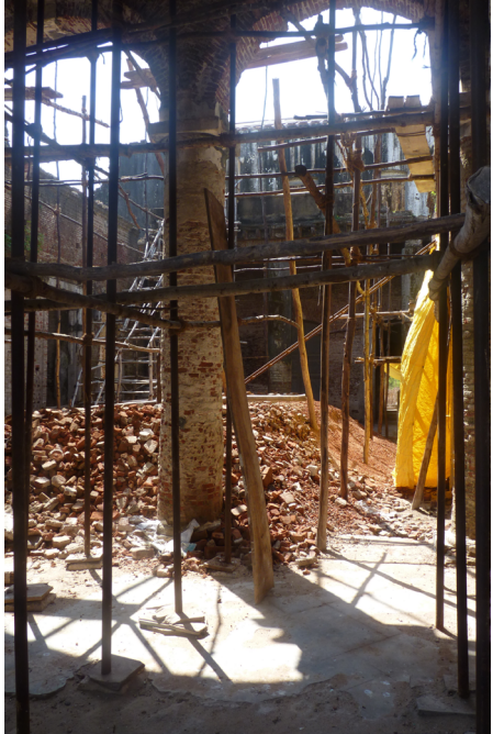
Fig. 7. Upper left: The construction system adopted for roofing and intermediate floors is known as the ‘Madras terrace’. The photo is showing the process of sticking bricks, starting in one corner of the roof.
