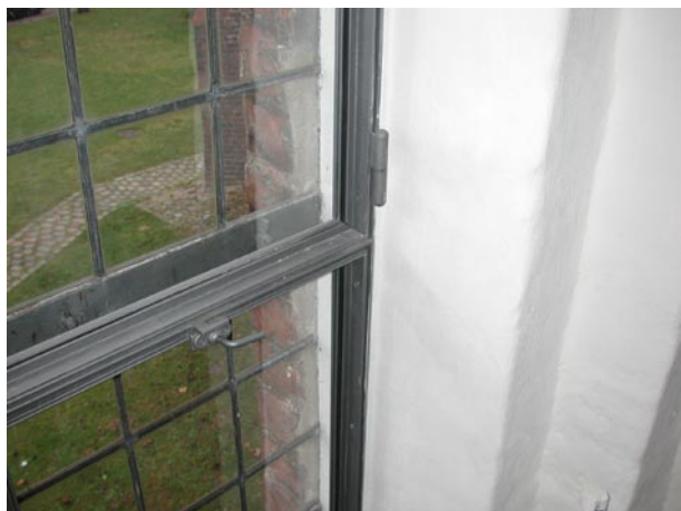
Figure 5. Detail of the windows in Sct. Olai church. The framing for the double glazing was custom designed to fit the original leaded windows. Photo by Poul Klenz Larsen
