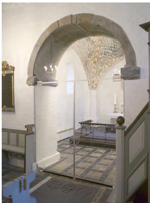
Figure 8. View through the glass door in the chancel arch at Dybe church. The lime painting in the vault is visible in the chancel. The heating elements on the wall below the vault are controlled by a hygrostat to keep the RH at 70-80% all year. Photo by Roberto Fortuna, the National Museum of Denmark.
